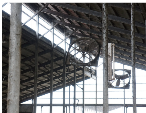
Ventilation of cowshed
